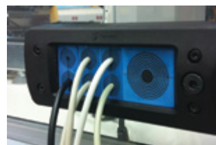
Roxtec sealed gland ports
